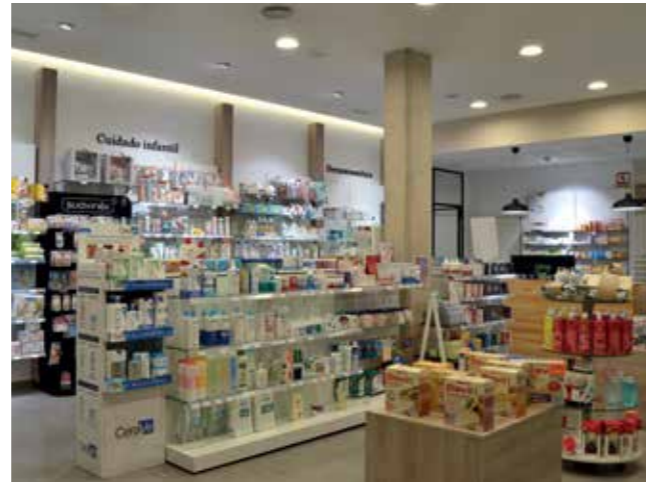
Compatible lighting with installations that require UGR<19
